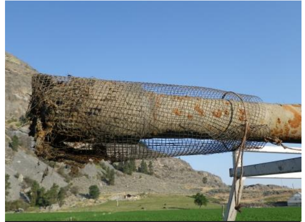
A set-up like this puts an irrigator at risk of regulatory action from WDFW.
