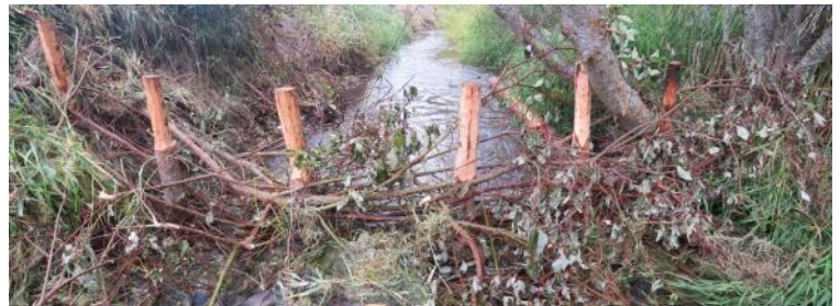
A beaver dam analogue: vertical pilings placed across the stream were woven with live cuttings to slow flows and to provide beavers with a stable starting place for dam building.
