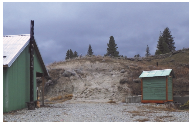
Erosion at the Tunk Valley Grange
