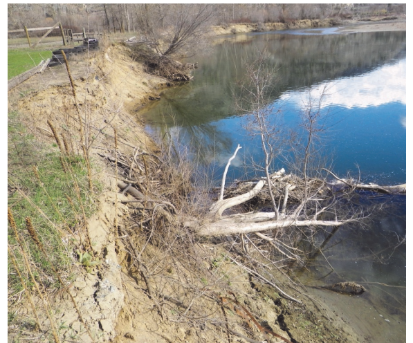
Okanogan River bank erosion
