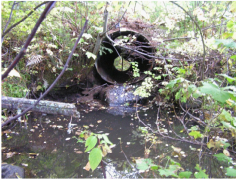
Existing 36" metal culvert which is a barrier as it is undersized for the stream and has an outfall.
