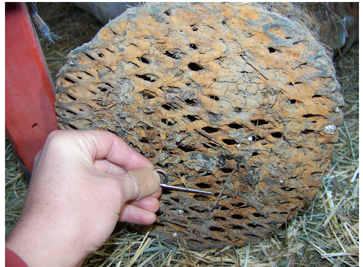
This screen greatly exceeds the opening standard and should be replaced.
